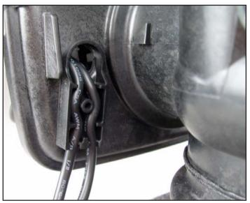
6b. Once each valve has all of the wires brought through the knock out on the backplate, you can then use pliers to break out each tab in the strain relief on the back. This will allow each wire to be weaved down on each.
